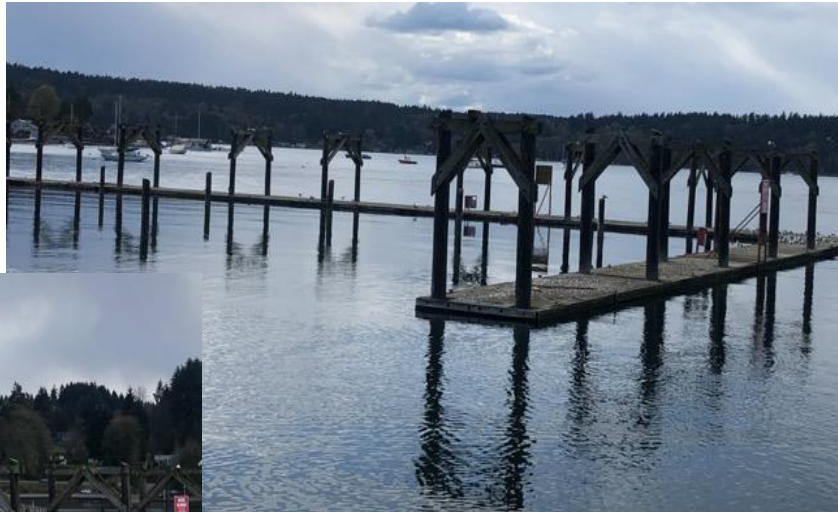
Dockton Progress – Only Inside Docks Removed
